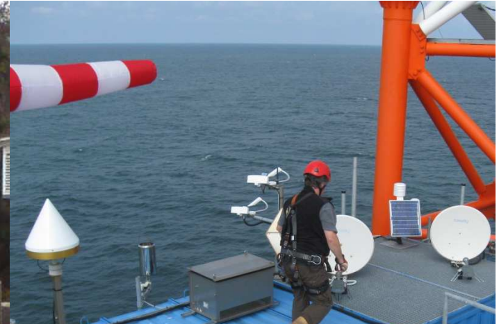
CL51 and Vaisala PWD52 on FINO3 platform
